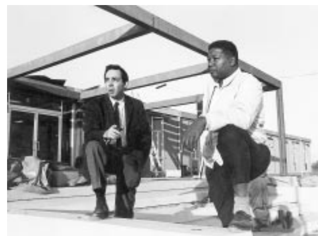
H. Jack Geiger, left, in 1966 on the construction site of the Delta Health Center on the outskirts of Mound Bayou, Mississippi. With him on what was formerly a cotton field is Dr. John W. Hatch, then the director of community organization and health education for the center. Photo, Dan Bernstein.
